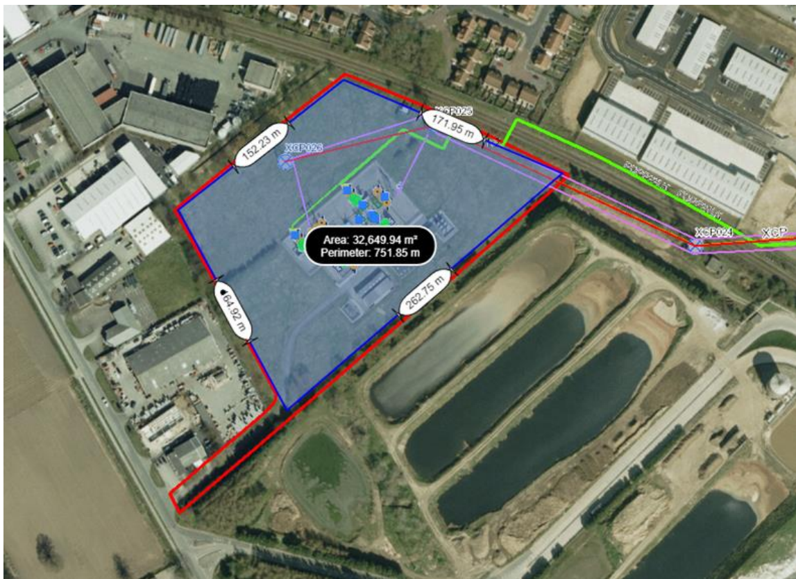
Figure 4.1: Existing Poppleton 275kV Substation (land ownership in red)
